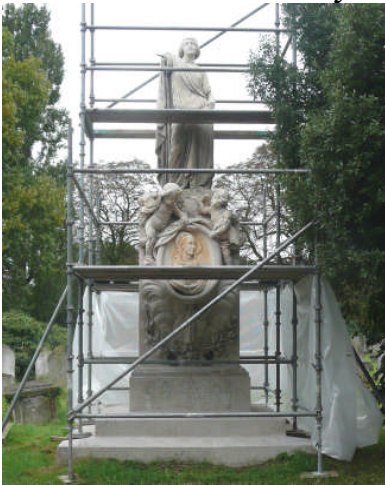
Soyer Monument during restoration Photograph by Mr Nicholas Mellersh
