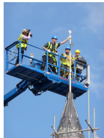
Re-installing the restored weathervane
