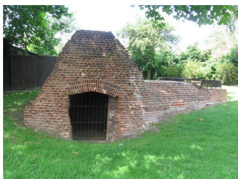
The Conduit Head after Restoration
