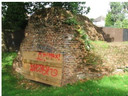
The Conduit Head before Restoration
